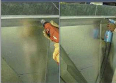
Riveting & Frame Fixing (4)
